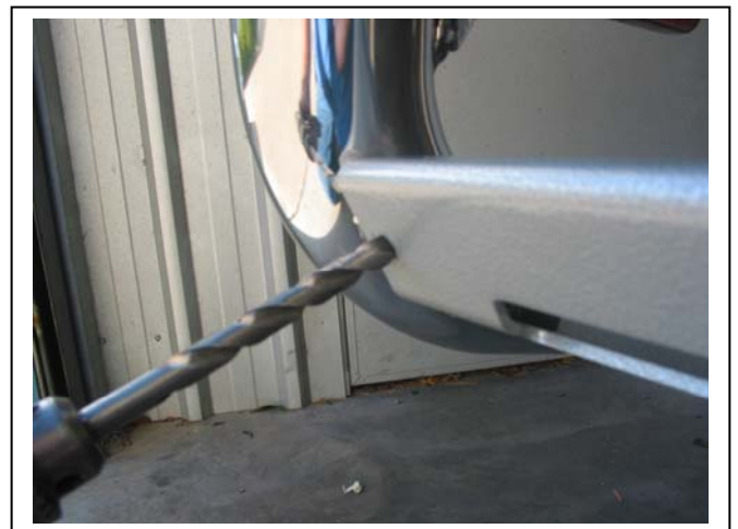
Figure 8: Drill lower holes to 10mm
